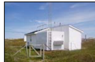
Figure 3: Atmospheric Chemistry building and storage shed on Sable Island. (Courtesy: Sable Island Green Horse Society).
